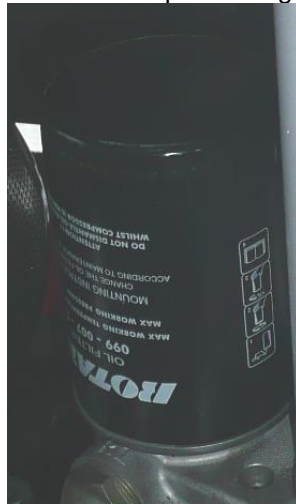
Figure 13.4-6 Compressor oil filter
